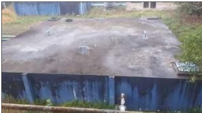
Gambar 3.44 Reservoir Air Serkuk II Kapasitas 300 m 3
