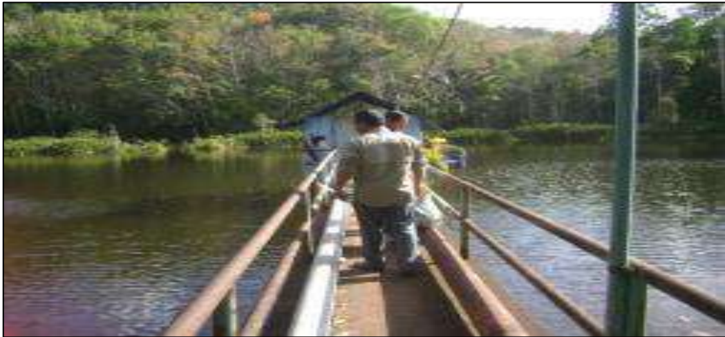
Sumber: Rencana Induk Sistem Pengolahan Air Minum (RISPAM) Kabupaten Bangka Selatan, 2015 Gambar 3-63 Kolong Baher & Intake (Unit Intake SPAM Baher)
